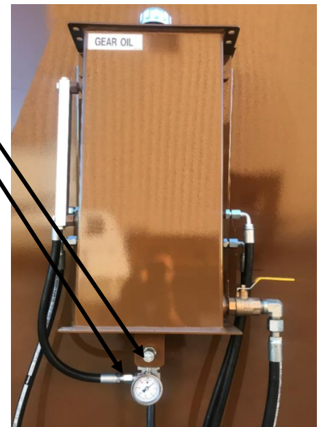
"T" gear box fill plug (full level)
